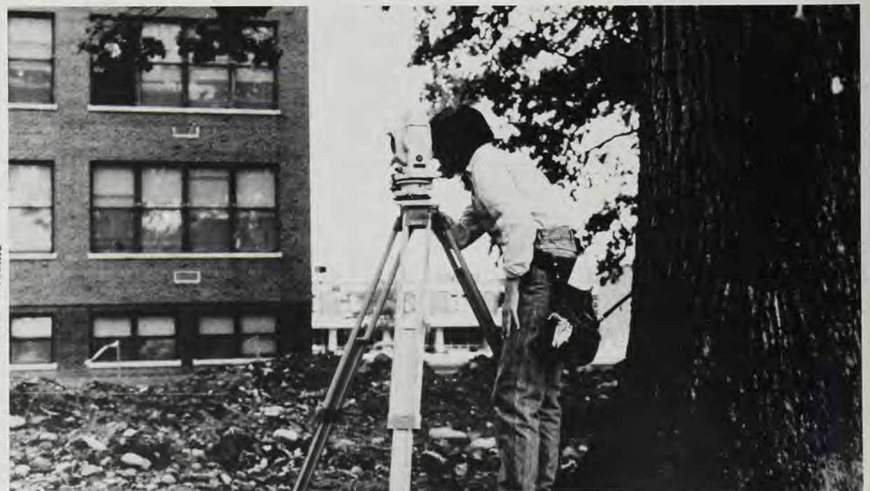
Surveyors check the level and distance.
