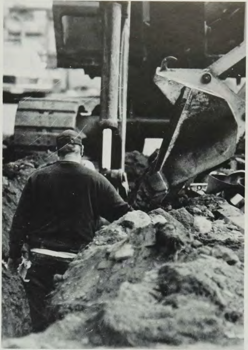
Heavy equipment dwarfs the workers.
